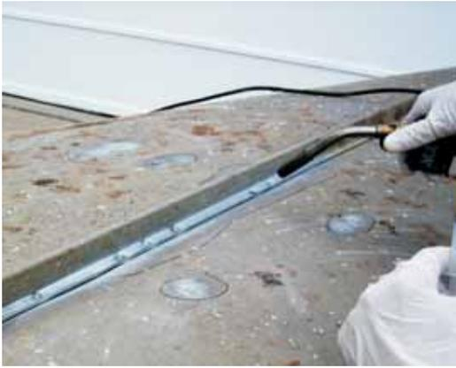
**Left—Clean the area around the leaky seams. Then heat the area with a propane torch to drive off moisture and warm the metal.**
