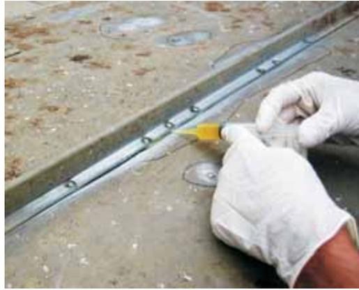
**Right—Force G/flex 650 into the seam with the syringe while the metal is still warm. Apply heat with a heat gun until the epoxy has gelled.**
