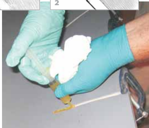
Injecting G/flex into a widened crack. Note paper towel in hand to clean up after rampant sloppiness.
